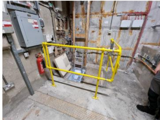
New edge protection to the ladder well
