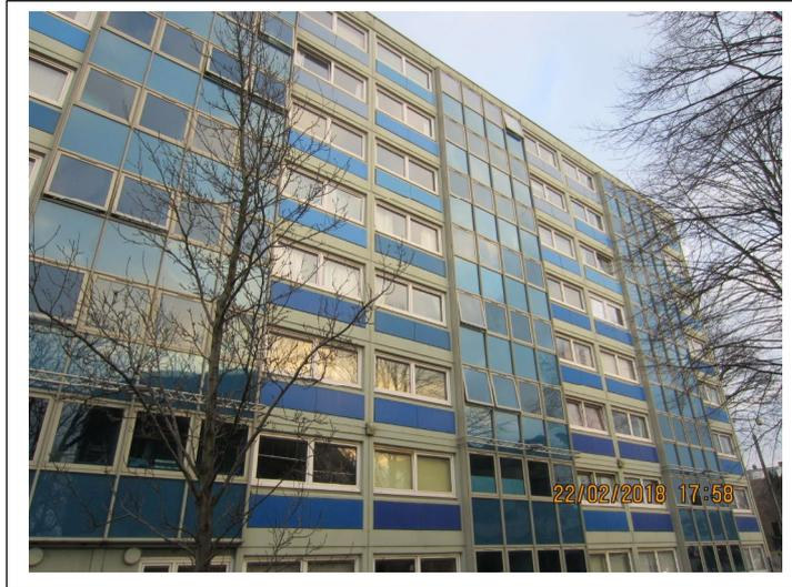
There is no cladding affixed to the external façade of the premises but there are additions to the original as-built façade. Specifically, curtain wall glazing and aluminium frames, fixed flush to the face of the concrete structural frame and panels, were fitted approximately 10 – 15 years ago to enclose a previously open balcony. The windows and doors between the living space and balcony area remain in-situ.
