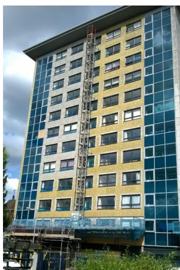
photos above showing the ongoing fitting of EWI and completed
