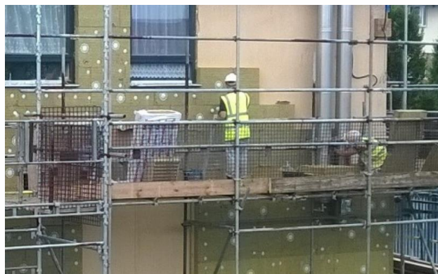
photos above showing the ongoing fitting of EWI and completed
