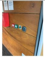
Certain final exit doors are provided with a sliding power assisted opening mechanism. Assurance was provided that these are linked to the fire alarm and open upon its activation. A 'Green Box' emergency override is also installed adjacent to the doors and opens the doors when activated.
