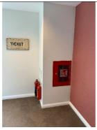
Firefighter dry rising mains are located in each block, so as to provide a firefighting facility due to the size and layout of the blocks. The inlets are located on the external façade and the outlets are located at each level of one of the staircases per block. The dry rising mains are subject to periodic service and inspection by a competent person, with records held centrally by WCHG.
