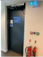
Final exits from the building are, in the majority, either electromagnetically secured with a suitable override or provided with push pad type opening devices.
